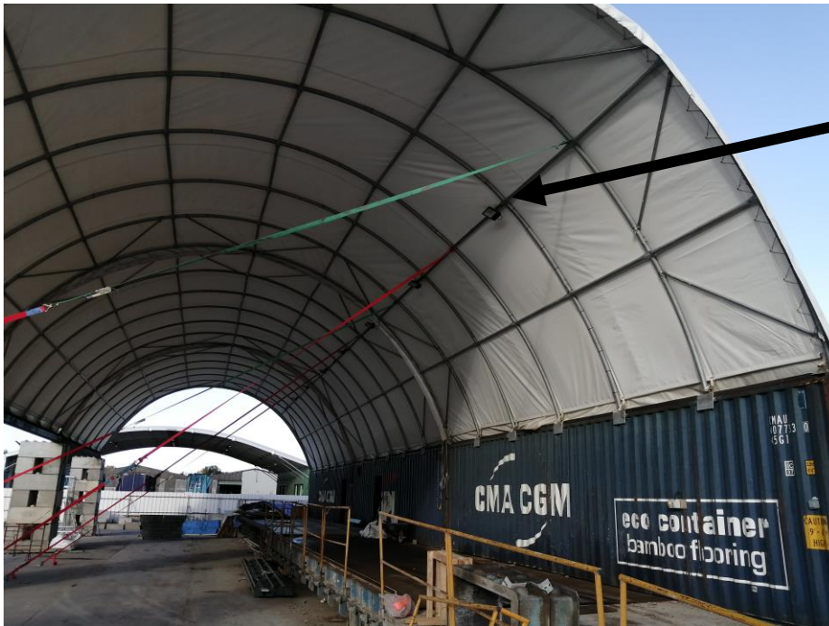
Existing lighting installed on site inside the structure
